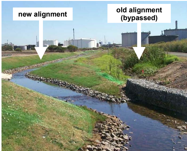
View of Springvale Drain from Mcpherson Street (downstream) end looking north
